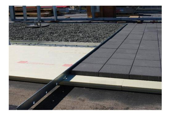
Commonly referred to as "upside down, *irma* or *prma* roofs" this method of insulated roofing simply means the insulation is placed above the waterproofing membrane and held in place by a specified ballast, usually river pebbles or concrete pavers.
