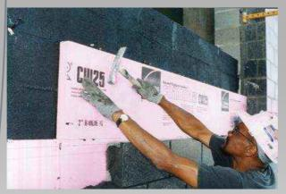
Foamular Extruded Polystyrene is closed celled insulation, so it is not effected by moisture. It can reduce the transfer of moisture and is its physical properties are not reduced in the presence of moisture.
