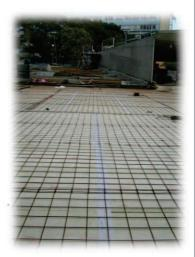
↑ Foamular Insulation at the University of Sydney, ready to have the slab laid on top.
