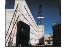
Insulated concrete panels are more comfortable than exterior concrete walls that are not insulated. Also, insulated panels help reduce heating and cooling costs by minimizing heat gain during the day and heat loss at night. With Herlong, Calif., located near the east side of the Sierra Nevada mountain range, there will be substantial temperature swings.
