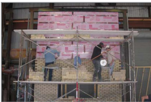
Figure 3: Test wall under construction
